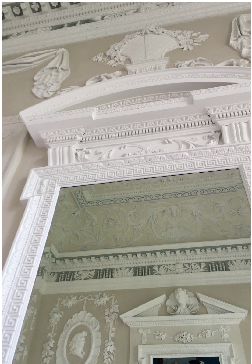
Fig. 6. Interior of Chatelherault, showing the restored ornate plasterwork. ©Amy Frost.
